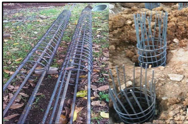
Gambar 2.7 Pondasi Strauss Pile
