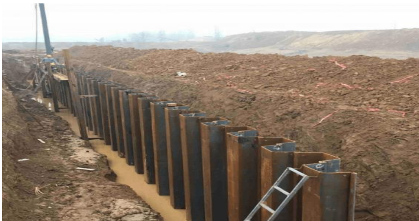
Gambar 2.6 Dinding Penahan Tanah Tipe Sheet Pile
