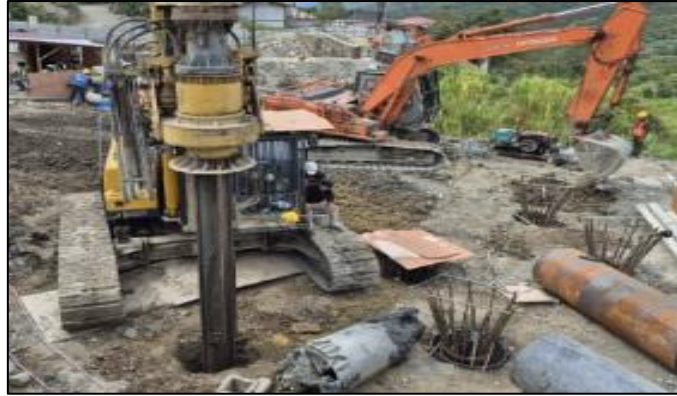
Gambar 2. 20 Pondasi Bore Pile
